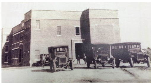
Early building (1925) still incorporated into the shoe factory today
