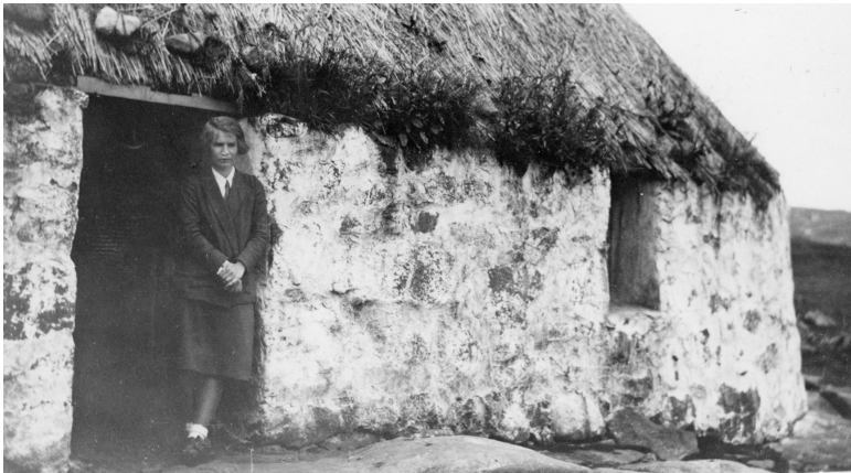
Margaret in the doorway of the MacRae's croft house
